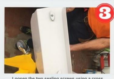
Loosen the two sealing screws using a cross screwdriver and an 8 mm hex key.
